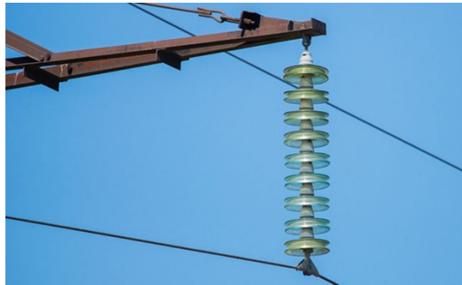
Figure 1: High-voltage insulator [3]
